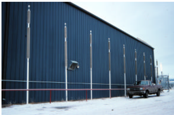
Figure 8. Thermosyphons used to cool the ground and prevent thaw subsidence of a building foundation, Northwest Territories. (Photo by R. Couture, 2000)
