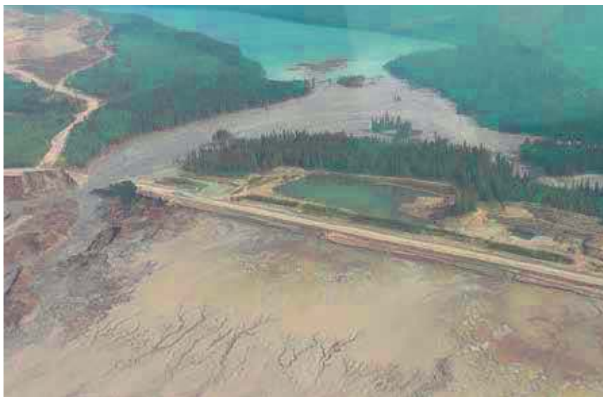
Morgenstern chaired the Independent Expert Engineering Investigation and Review Panel for the Mount Polley tailings storage facility after the August 4, 2014, failure in British Columbia. (Photo: Reuters.)
