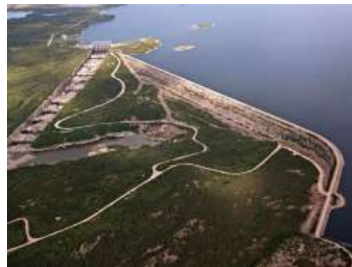
La Grande-2 main dam and spillway.
