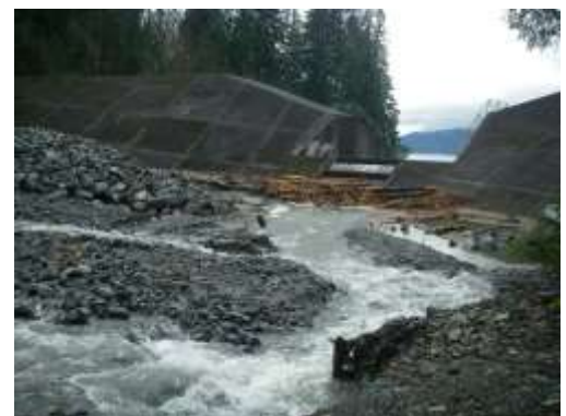
Structure after 2009 debris flow, and before debris was removed (for scale, the width of spillway opening is ~8 m).
