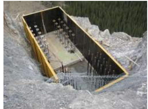
North footing during construction showing micropiles and extensive rock anchors.
