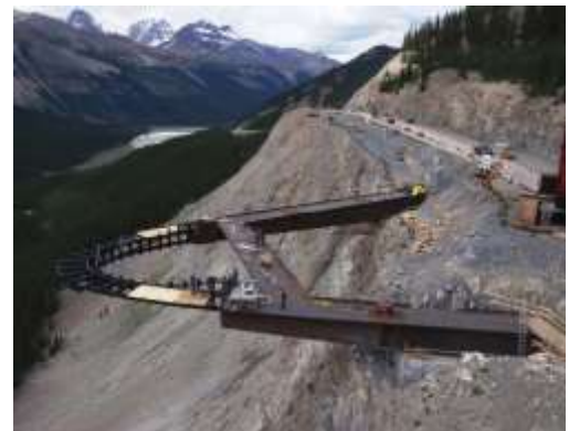
Aerial view during construction showing large footings and steep rock slope.
