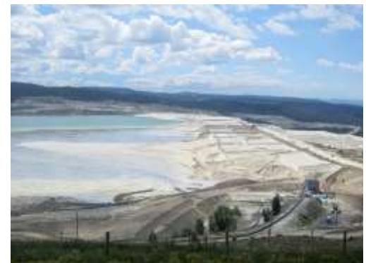
Upstream cyclone sand cell construction at the L-L Dam.
