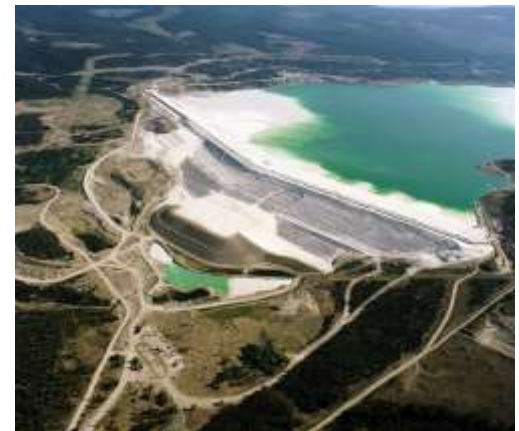
166 m high L-L Dam at north end of tailings facility.
