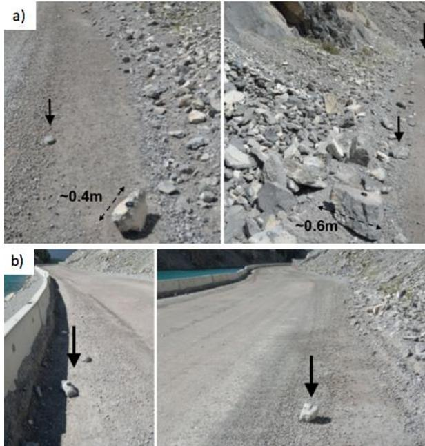
Figure 5. Fallen blocks found adjacent to the highway at the toe of the talus slope in sector F (a) and east of the road, adjacent to the barrier at the lake side (b)
