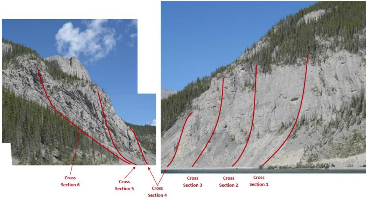
Figure 11. Cross sections selected for run out analysis of fallen debris
