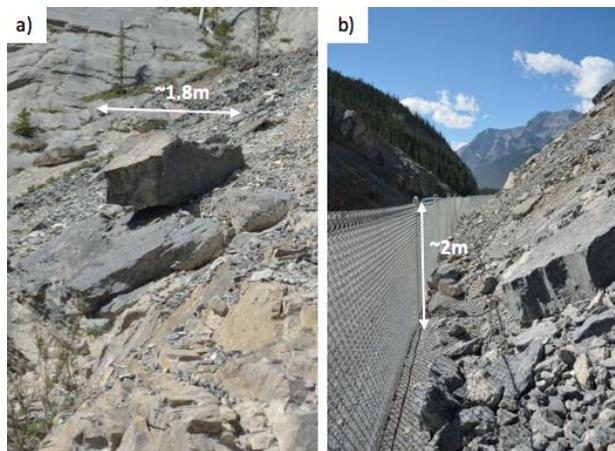
Figure 4. Rock blocks larger than 1 m<sup>3</sup> contained within the talus slope at sector C in Figure 2 (a) and adjacent to the road at sector D (b)
