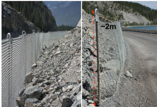
Figure 6. accumulation of rock debris contained by existing 2m-high fence at sector D and E in Figure 2
