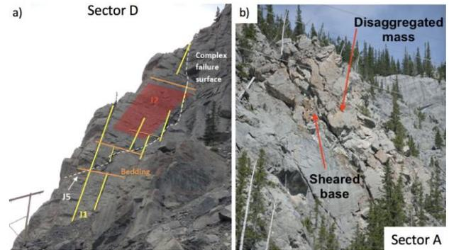
Figure 7. Evidence of progressive failure mechanisms that can lead to larger failure volumes
