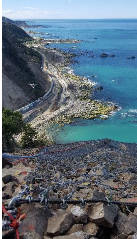
Figure 6: Completed drape showing perimeter anchor connection detail
