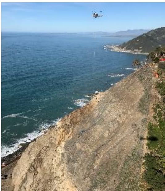
Figure 5: Helicopter installation of the ring net
