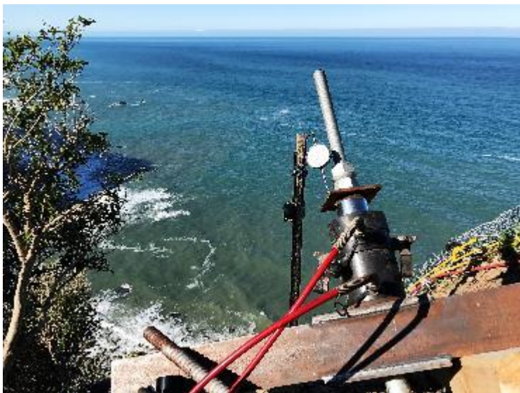
Figure 4: Acceptance testing of the perimeter anchors.
