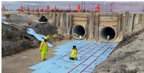
Figure 2. Rigid insulation placement at site 3
