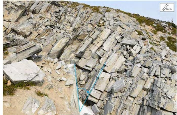
Figure 17. Mount Currie: Field photograph of a disturbed rock mass in area no. 2 of Figure 15 (from: BGC Engineering report).
