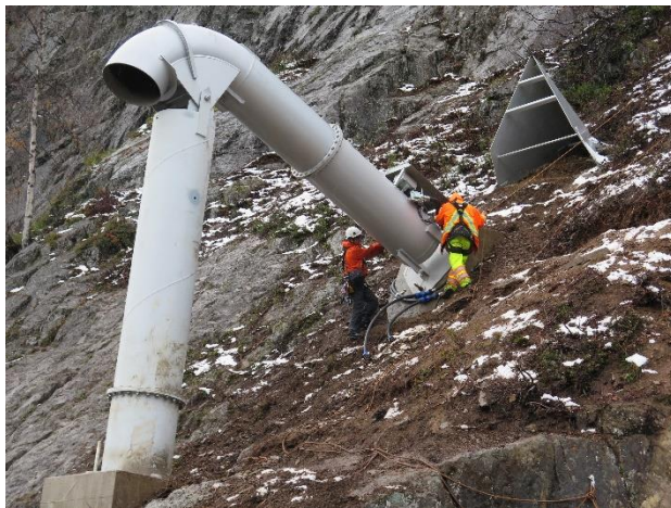
Figure 17. Gazex ® gas-based RACS. As of 2017, there are six Gazex exploder installations in paths affecting the TCH, approximately 10 km west of Lake Louise
