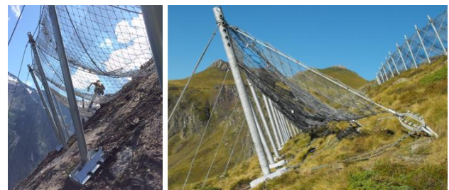
Figure 7. Geobruigg SPIDER snow net floating base plates.
