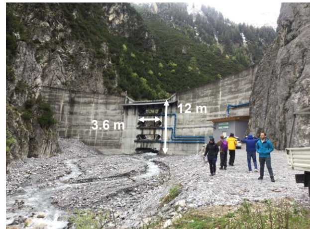
Figure 6: Debris-flow barrier on Schnannerbach in Austria. Photograph by E. Moase, May 2016.
