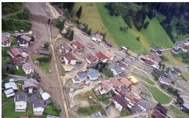
Figure 2: Debris-flow damage on Schallerbach following the June 2015 event. Photograph by Feuerwehr Landeck .
