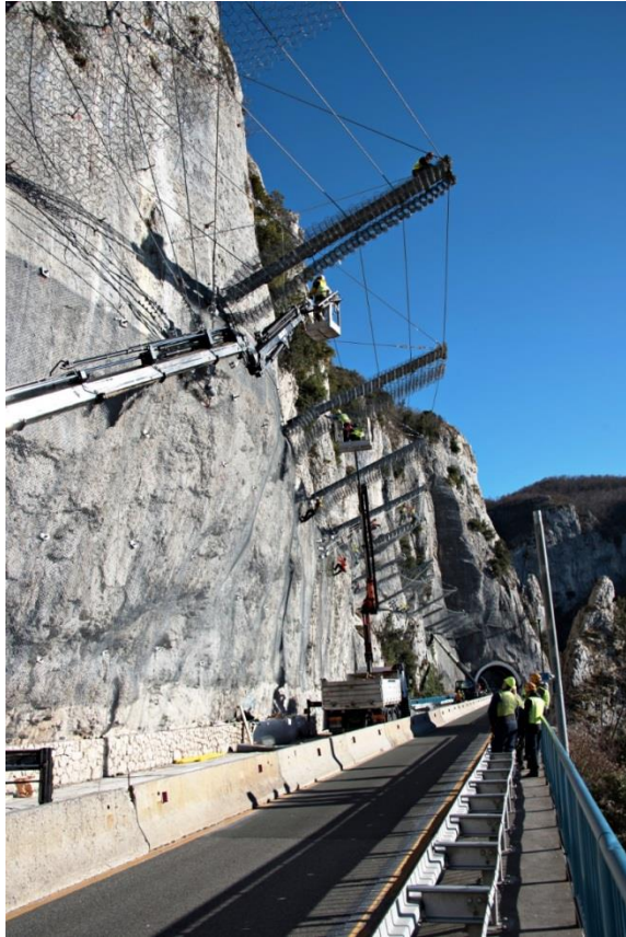
Figure 6. Installation of the 3000 kJ rockfall fence.
