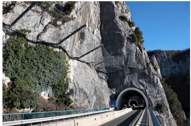
Figure 7. Complete portal protection (left: western portal, right: eastern portal)
