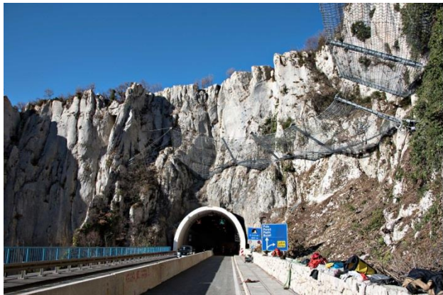
Figure 7. Complete portal protection (left: western portal, right: eastern portal)
