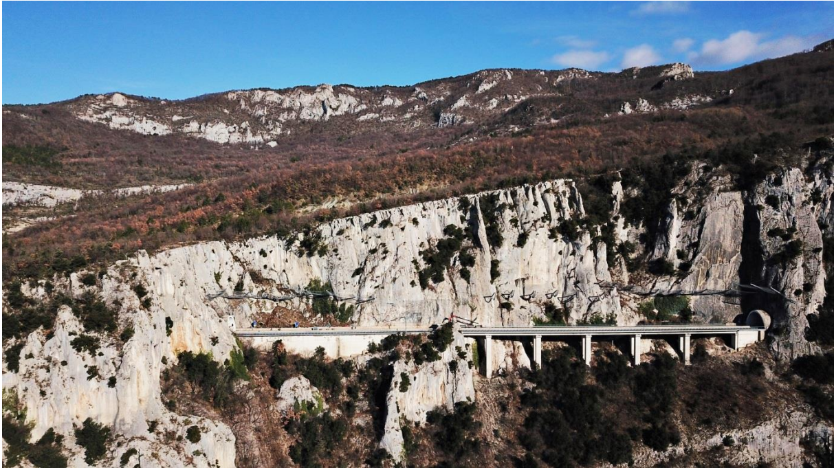
Figure 3. Oblique aerial view of project site showing partially installed mitigation measures.
