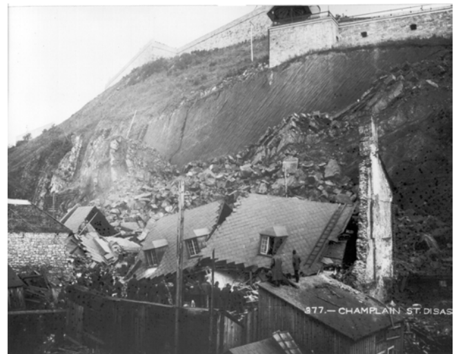
Figure 3. Contemporary photograph of the September 1889 Champlain Street landslide disaster, Québec, Québec. 50 people were crushed to death in the houses at the base of the failed rock slope, below the walls of the Citadel. (Public Archives of Canada Photograph 131073).
