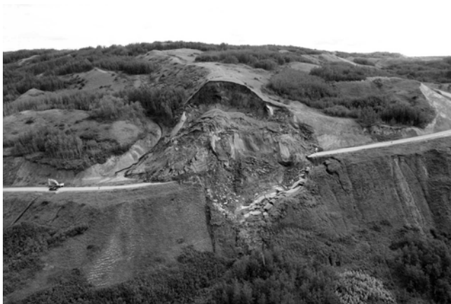
Figure 14. First phase of landslide in glaciolacustrine silts and clays, Beaton River valley, near Fort St. John, B.C. (Raymond et al., 2003). The landslide severed BC Road 103 in 2001 interrupting agricultural and oilfield traffic. Soon after this photograph was taken, the landslide developed into a more complex failure (photograph courtesy of BC Ministry of Transportation and Highways).
