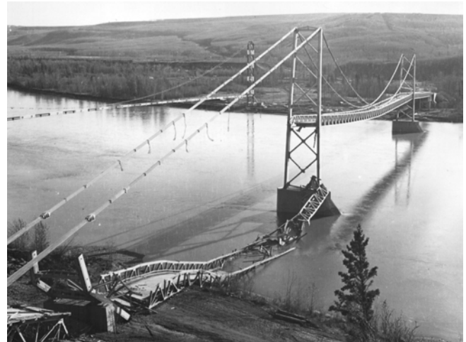
Figure 15. The 1957 collapse of the Peace River Bridge, Alaska Highway, Taylor, British Columbia, caused by sliding of the north anchor block (left foreground) in Cretaceous bedrock (photograph courtesy of the North Peace Historical Society).
