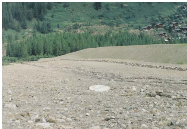
Figure 8: A diversion berm in Switzerland used to reduce the risk of destructive avalanches spreading into the developed area beyond. C. Stethem photo.
