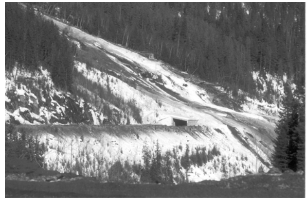
Figure 3: Avalanche over a snowshed on the Trans-Canada Highway near Rogers Pass, BC. C. Stethem photo
