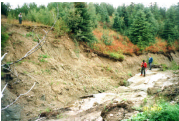
Figure 11. Photo showing the depth of the washout at the original road crossing. Note persons for scale.
