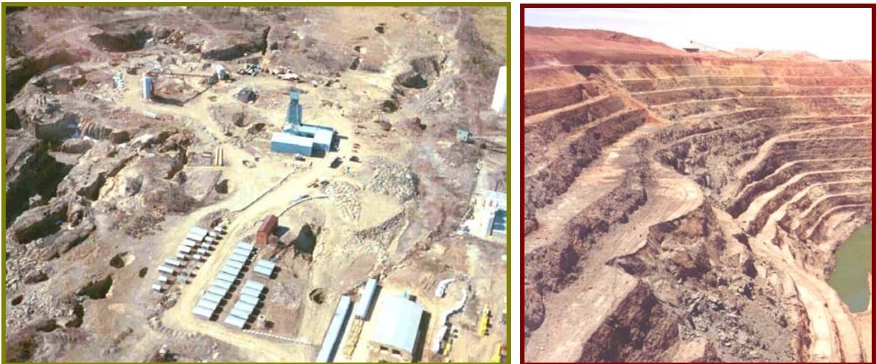
Figure 1: Ground movement associated with: 1) mine subsidence, and 2) mine pit wall instability.
