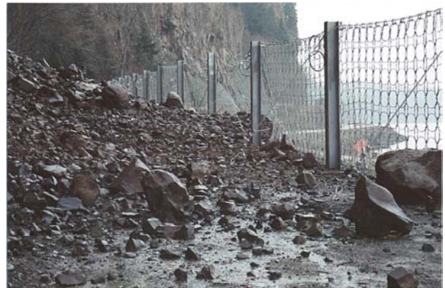
Figure 9. Rockfall Barrier impacted by rock slide
