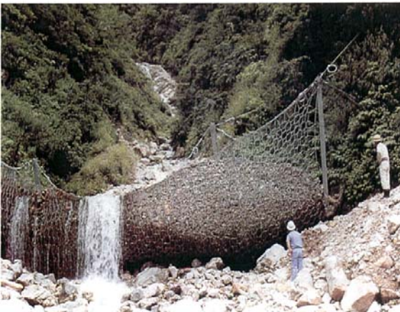
Figure 13. Debris flow of approx. 720 m 3 stopped by flexible barrier in Japan
