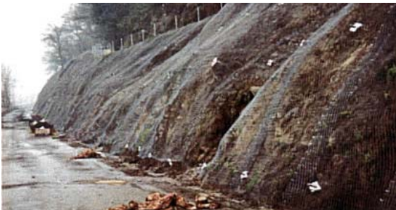
Figure 16. High strength mesh anchored to slope
