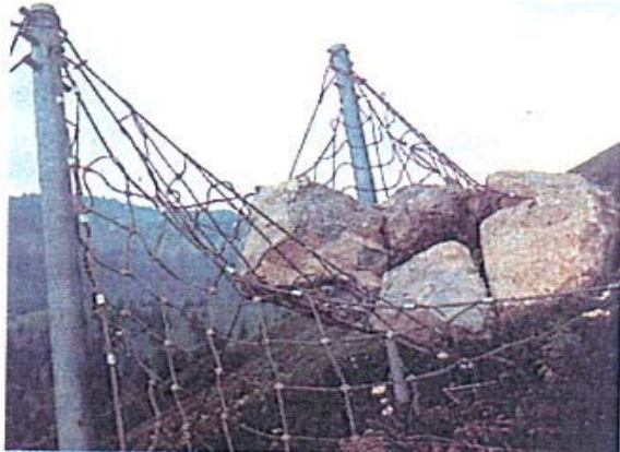
Figure 4. Rock impact to avalanche prevention structure
