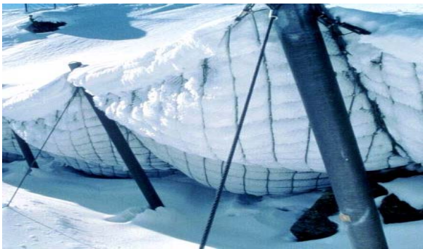
Figure 1. Wire rope net supported by steel posts
