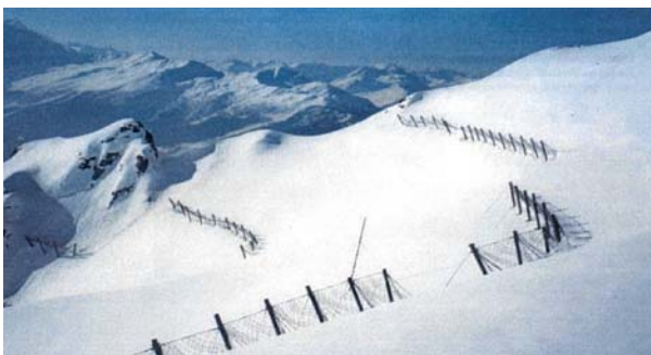
Figure 2. Series lay-out of avalanche netting structures
