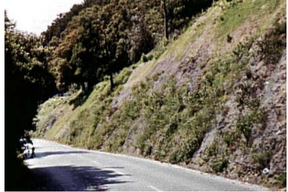
Figure 17. Re-vegetated slope after mesh installation
