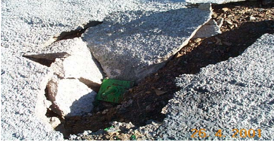
Figure 15. Shotcrete cracked at anchor point
