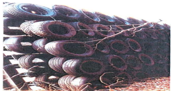
Figure 3. Rubber tire rockfall barrier.
