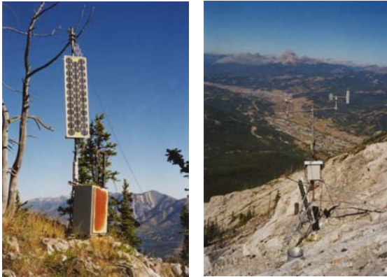
Figure 8. Seismic station (left) and weather station (right) near the summit of South Peak (BGC 2000).
