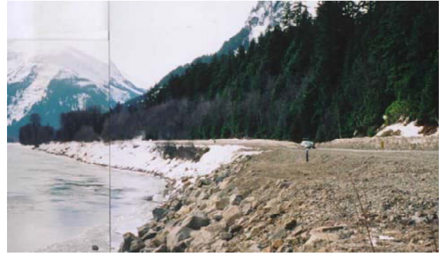
Figure 12: View looking downstream after site investigations and February bank repair. (The slope inclinometer casing in the photograph is near the upstream edge of the backscarp).
