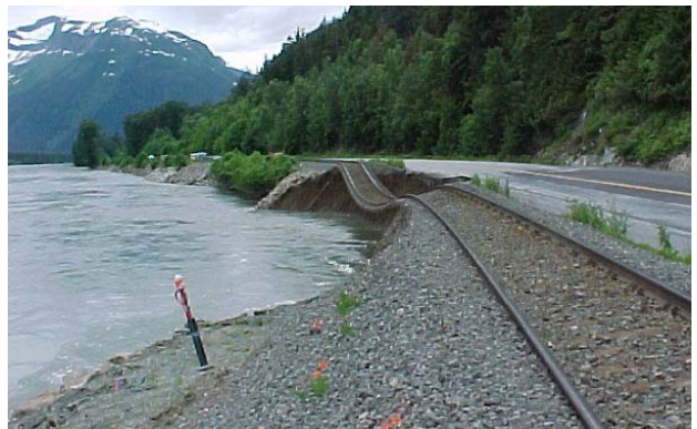
Figure 13: Skeena Mile 28: View looking downstream at July 18 landslide site
