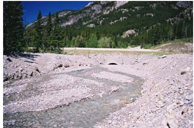
Figure 9 – East channel downstream of the highway culvert in September 2002. Note the large quantity of gravel in the channel compared with Figure 6.
