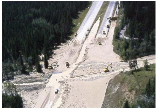
Figure 1 – Immediately after the August 1999 debris flow, clearing the Trans Canada Highway (photo courtesy of Parks Canada)
