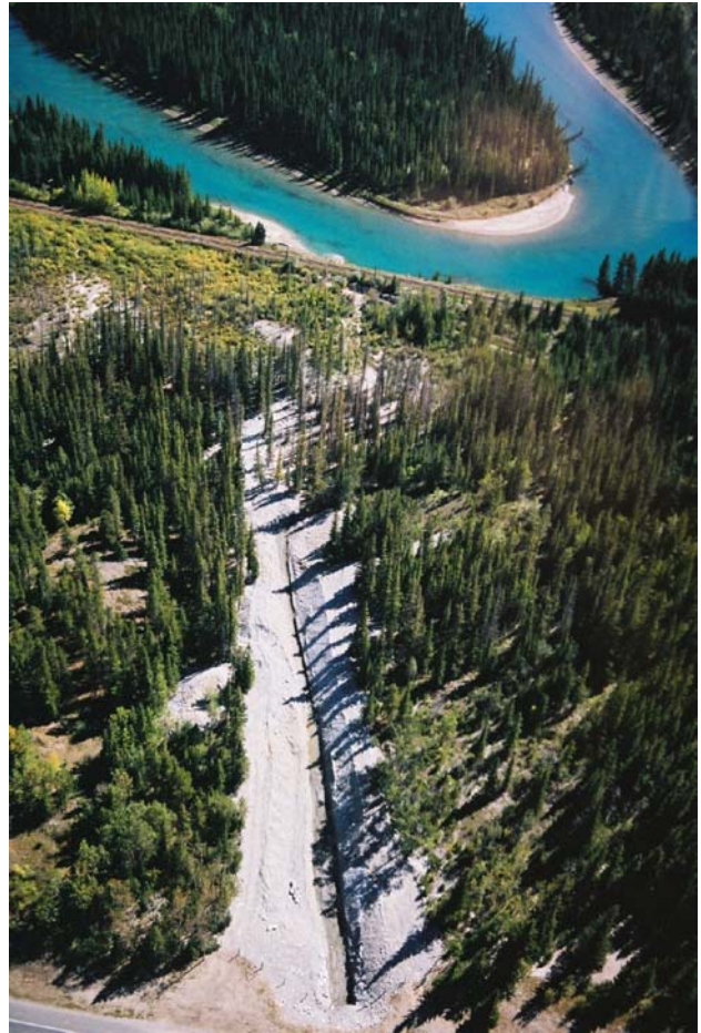
Figure 7 – Lower portion of the east channel towards the Bow River. The channel has been cleaned several times.
