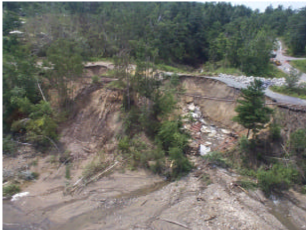
Figure 5. Oblique aerial photo of one of the many massive-shear subgrade landslides and seepage erosion sites near Port Kent (north of Port Douglas, NY).
