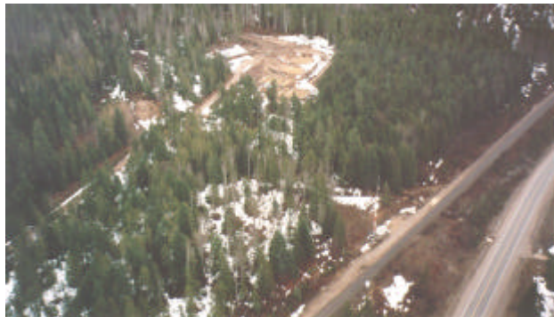
Figure 4. Oblique aerial photo of Shuswap Sub, Mile 22.6 on April 4, 1999 following a debris slide into the Fish Hatchery during the spring of 1999. This event did not affect the railway or highway. The June 13, 1990 debris flow inundated the track immediately east (right) of the radio tower.
