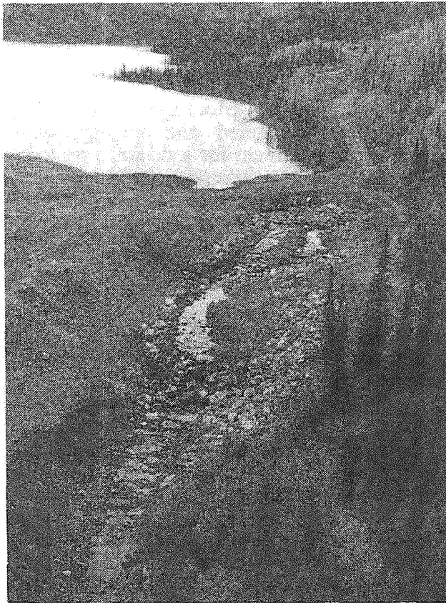
Photo 3: View of the Hudson Lake outlet and armoured channel.
