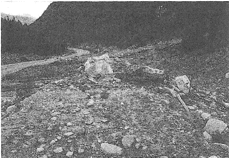
Plate 3. Same location as Plate 1 showing debris torrent deposits on top of a 6.2 m high berm located downslope of the Lightguide right-of-way. Debris flow deposits in the background covered the Lightguide to a depth of at least 2 m. (April 29, 1991)
