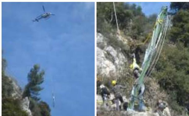
Figure 13. Installation of the barrier post using helicopters.
