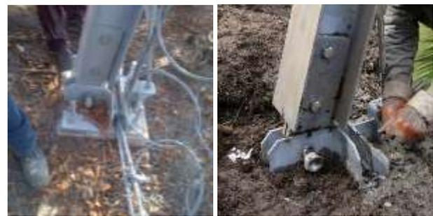
Figure 14. Example of post base systems. Left: a small concrete plinth has been realized to give a flat base to the post. Right: the base plate is directly installed on the ground.
