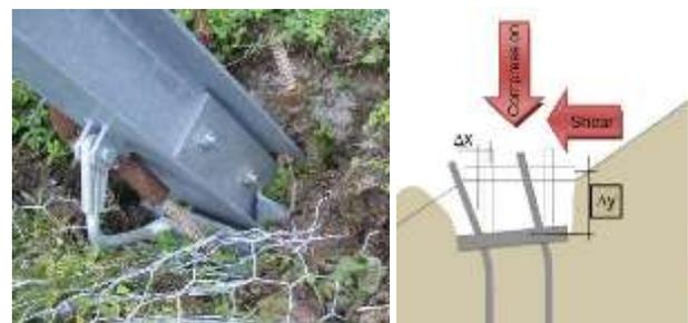
Figure 15. Settlement of the footplate after the impact. The vertical ( $\Delta y$  = approx. 200 mm) and the horizontal ( $\Delta x$  = approx. 50 to 100 mm) displacements of the base plate represent a benefit for the energy dissipation of the fence.
