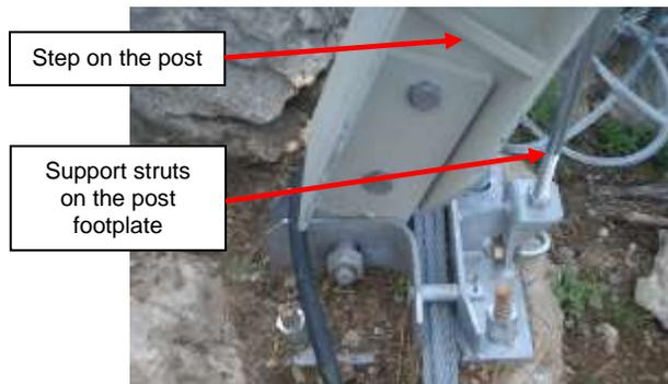
Figure 12. Example of devices to help the installation: steps on the post and support struts on post footplate.
