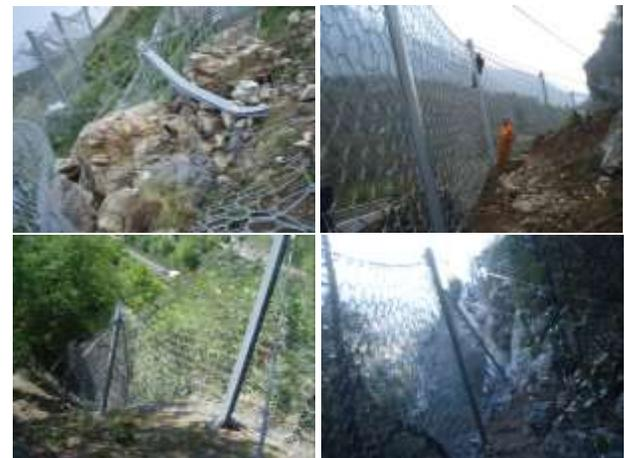
Figure 10. Examples of installed barriers. Top-left: barrier impacted by several blocks in different part of the fence. Top-right: barrier longer than 30 m with upslope concavity. Bottom-left: barrier with posts placed not at the same level. Bottom-right: barrier with posts installed without the same inclination.
