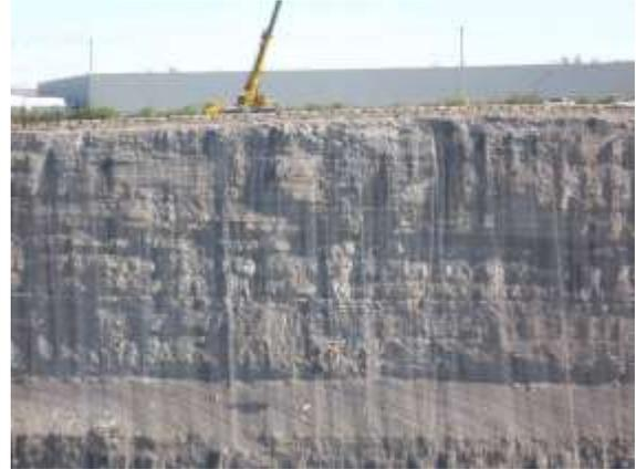
Figure 16. General front view of the rock slope where more than 40,000 m<sup>2</sup> of SteelGrid were installed in 2012 (courtesy of CIMOTA Inc.).
