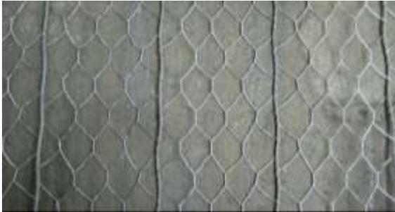
Figure 14. Detail of the cable woven in the double twist mesh to form the SteelGrid (in this example the cables are woven every 30 cm to reach very high performances).
