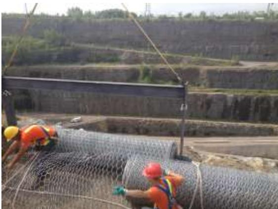
Figure 15. Detail of the installation of the mesh around the suspension cable at the top of the rock cut (courtesy of CIMOTA Inc.).
