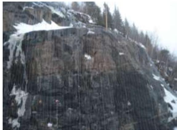
Figure 5. Simple drapery system at Manic 2 (Québec, Canada). Average height of the slope approx. 40 m, surface approx.  $5,000 \text{ m}^2$ .
