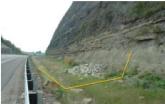
Figure 3. Example of a simple drapery mesh with a ditch (highlighted with the yellow line) at the base to collect the debris falling from the slope.
