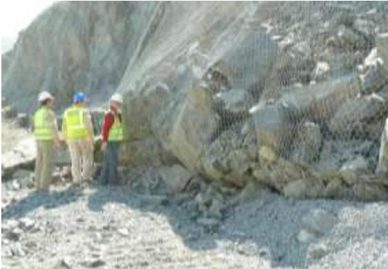
Figure 2. Debris and rock piled up at the bottom of a simple drapery system fixed at the toe of the slope by anchors and a down-slope longitudinal cable.
