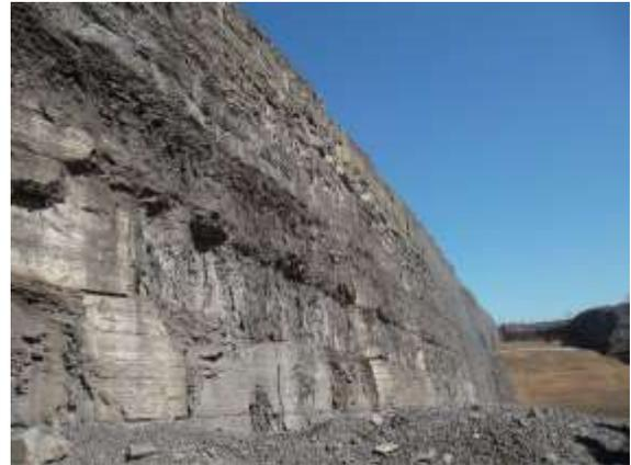
Figure 13. Front view of one of the rock slope at quarry Démix, before the installation of the rockfall mitigation system (average height of the cut approx. 120 m) (courtesy of CIMOTA Inc.).
