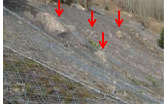
Figure 4. Example of a simple drapery system with cable panels and double twist mesh. The weight of the mesh (approx.  $5.0 \text{ kg/m}^2$ ) can avoid the rolling of single boulders (red arrows) along the slope.
