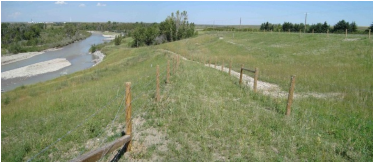
Figure 7. Facing north at the main buttress fill area in August 2013, showing the benched fill slope and livestock access path with vegetation becoming well-established.
