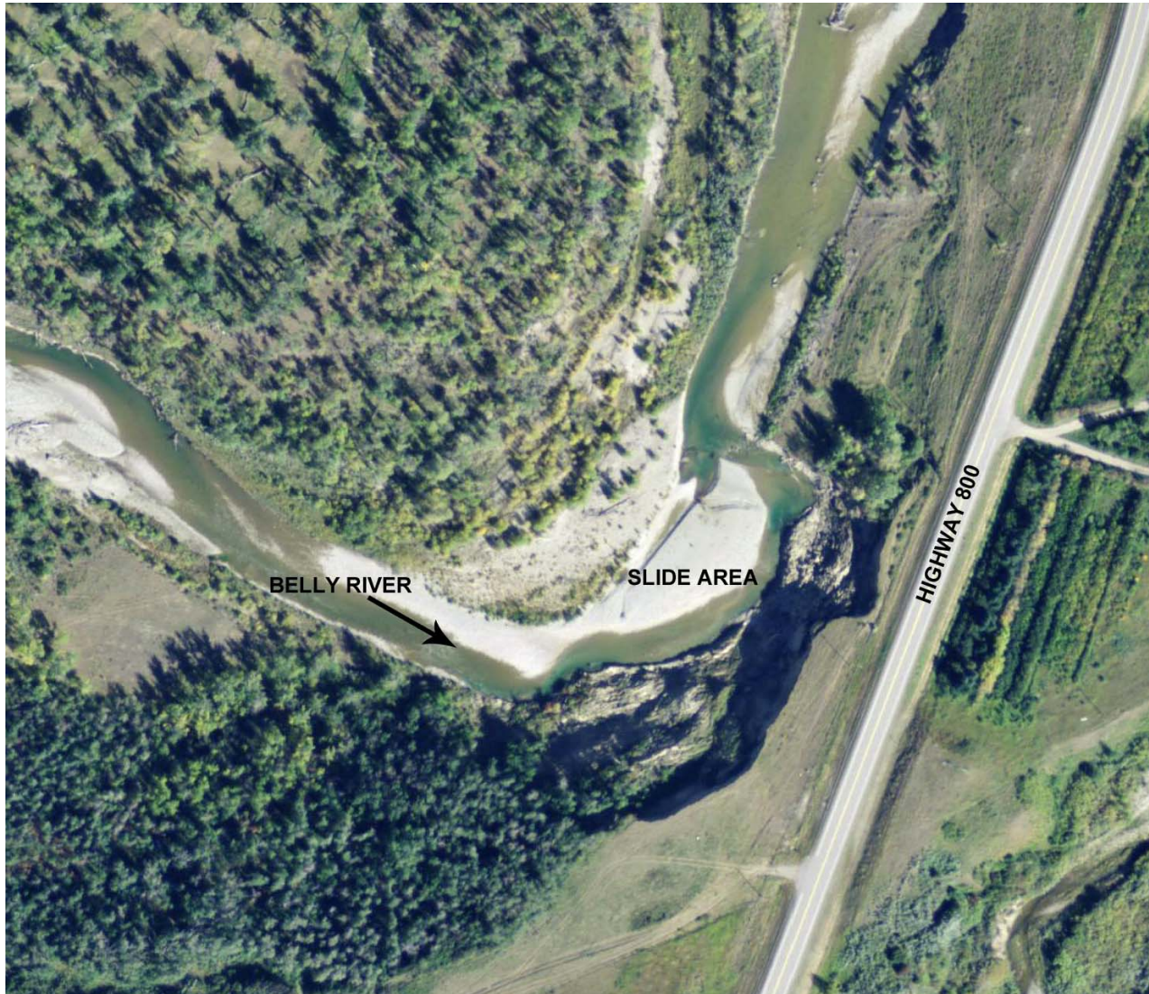
Figure 3. Aerial image of the site area in 2009.
