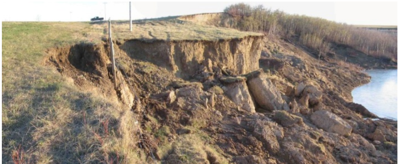
Figure 2. Facing south at the area of main slide encroachment in May 2010. The highway embankment is visible at the left edge of the photo. Block topples and rotational or flow landslides are caused by river erosion and groundwater seepage.
