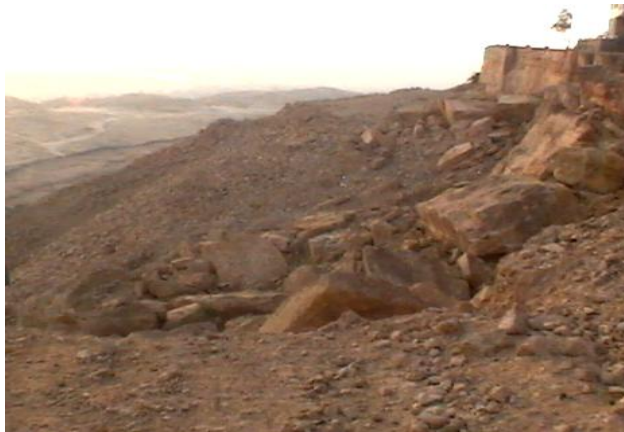
Figure 5. Endangered building due to slope failure
