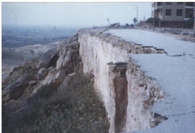
Figure 6. Road collapse at the western edge of Plateau
