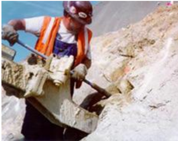
Figure 13. Rock Anchor on slope face
