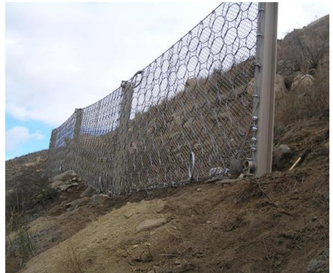
Figure 12. Catch fence of wire-ring net near slope toe
