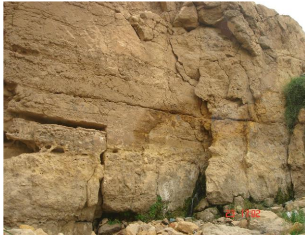
Figure 7. Seepage through rock cracks
