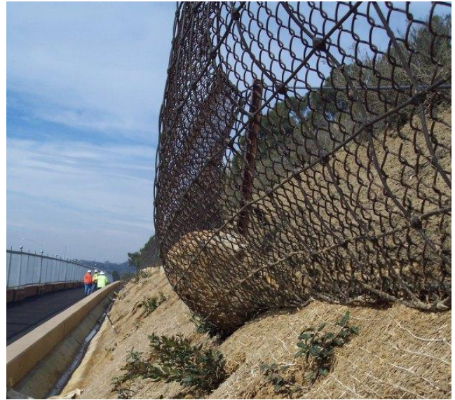
Figure 11. Guard mesh protecting road from rockfall
