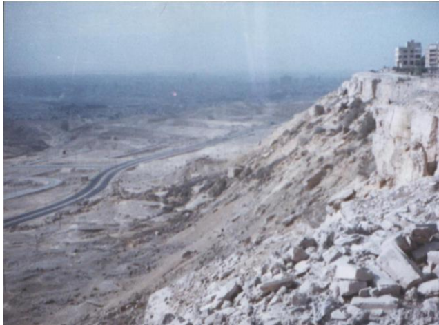
Figure 2. Rockfalls along the western cliff
