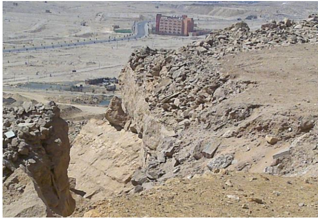
Figure 4. Newly detached rock mass at Mokattam cliff
