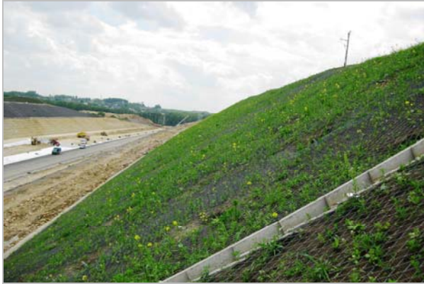
Figure 1. Slope stabilized with high-tensile strength steel wire mesh
