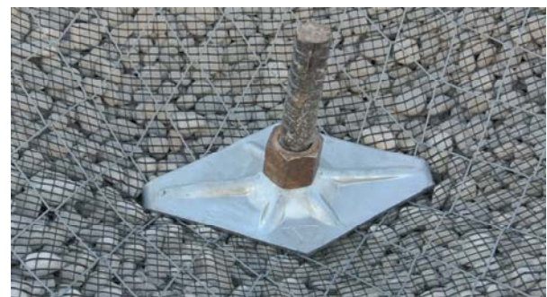
Figure 3. Spike plate type P33 (300 x 190 x 7 mm)
