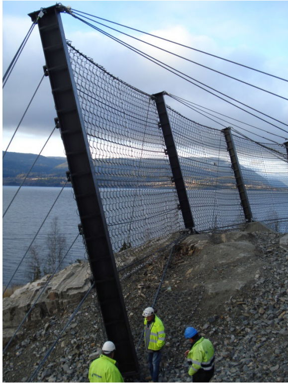
Figure 11. Varying height of posts to adapt to topography.
