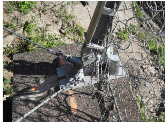
Figure 5. Adapted base plate for floating foundation.
