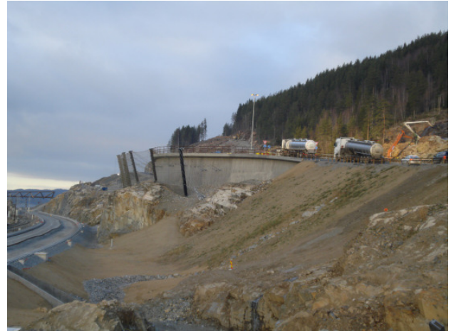
Figure 10. Rockfall catchment used for preventing vehicles from landing on railway (photo courtesy of Marco Toniolo, Pfeifer Isofer).
