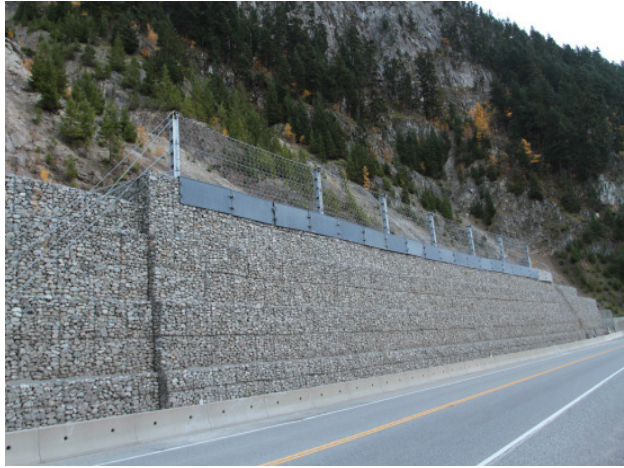
Figure 2. Fixed-rotation system installed on a double-sided MSE wall.
