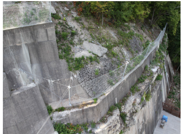
Figure 4. Floating rockfall catchment fence on pre-existing concrete wall.
