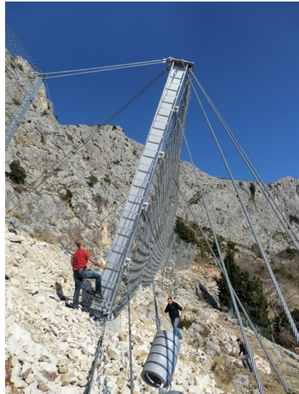
Figure 1. An example of an 8.5 m high post that exceeds the allowable height under current guidelines.
