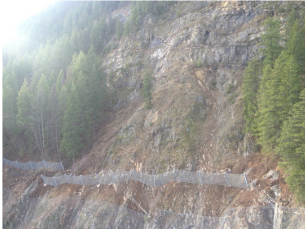
Figure 8. Rockfall catchment fence crossing avalanche path (photo courtesy of Jim Guinn, Mountain Rock Stabilization).
