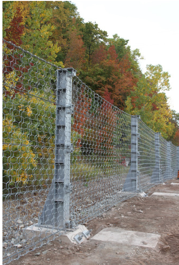
Figure 7. Reinforced catchment fence with additional middle bearing ropes.
