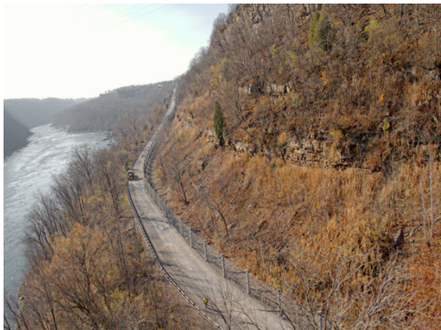
Figure 6. Fixed-rotation rockfall catchment fence installed at edge of access road.
