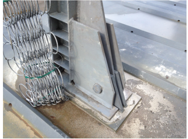
Figure 3. Adapted base plate for connection to foundation.
