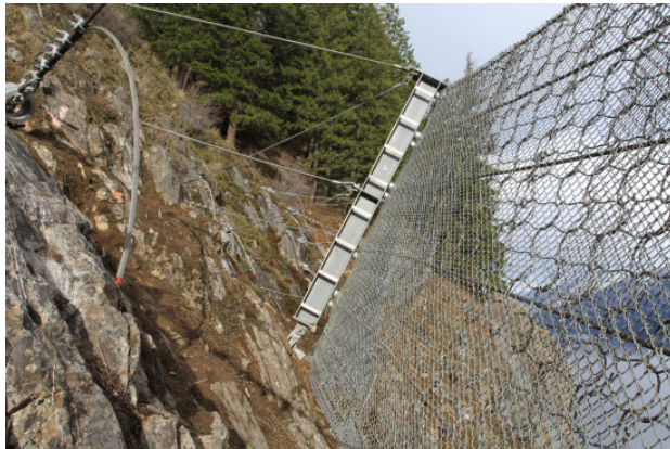
Figure 9. Reinforcement of post using retaining ropes connected at mid-height.
