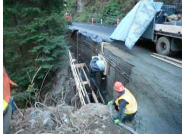
Figure 16 - Lost Creek wall complete with new asphalt ready for shotcrete.
