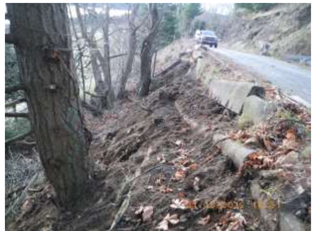
Figure 12 - Preliminary grubbing completed. Barrier and logs exposed.
