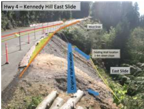
Figure 6 - Kennedy Hill East Slide pre 2011 construction
