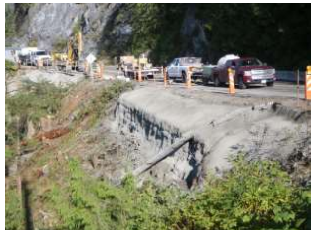
Figure 4 - Kennedy Hill West Slide complete.
