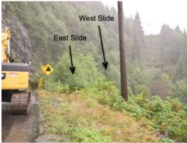
Figure 5 - Typical West Coast Terrain and the site of the Kennedy Hill East and West Slides
