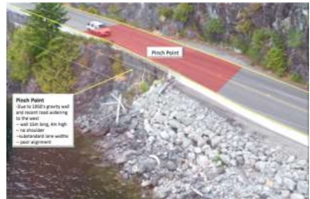
Figure 8 - Kennedy Hill Pinch Point overview
