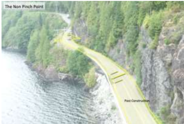
Figure 10 - Completed works with additional 2m of width
