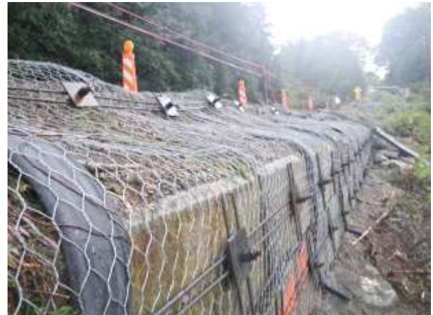
Figure 3 - Tie back soil anchors through the 2008 concrete blocks and shoulder fill, pre shotcrete.
