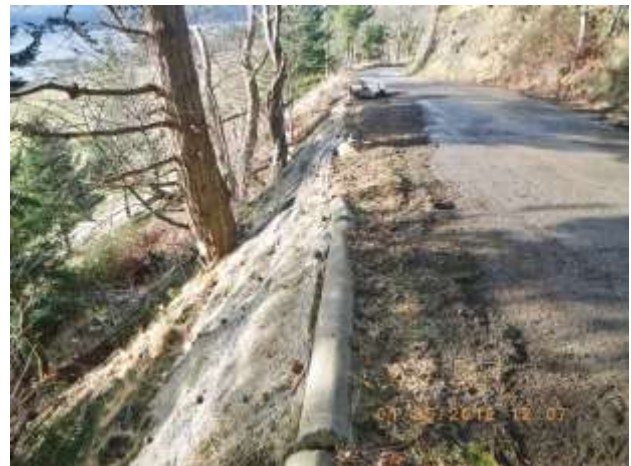
Figure 13 - Completed project using loose straw for revegetation, wire mesh facing with closely spaced soil/rock anchors.
