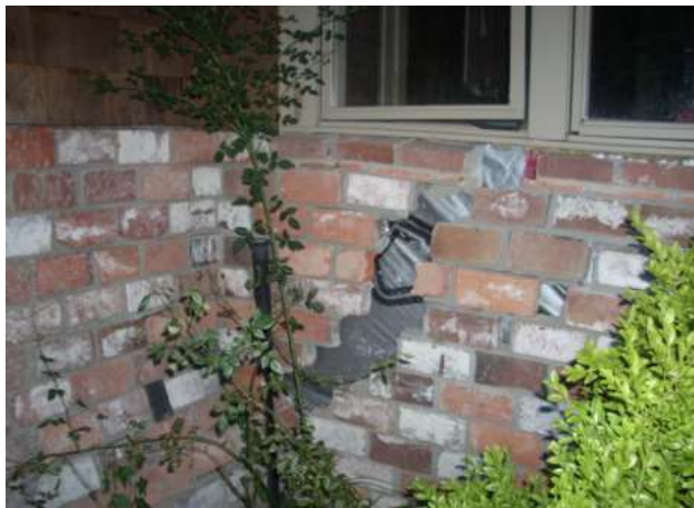
Figure 3 Example of damage to existing residences caused by ground movement (Watts 2010)
