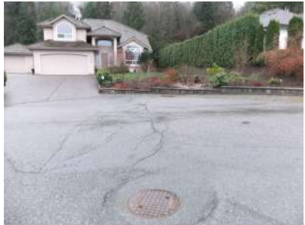
Figure 4 Example of damage to pavement caused by ground movement
