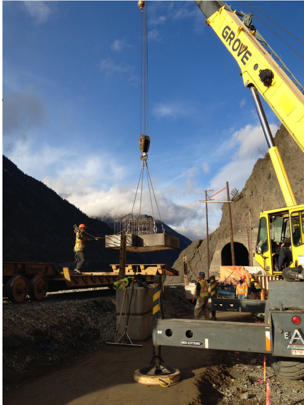
Figure 5 Installing one piece of pre-cast concrete footing along the upstream side of the rock shed.
