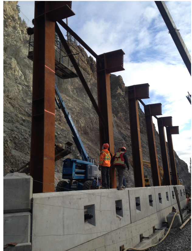
Figure 6 First row of modular pre-cast concrete panels tied back to the bedrock with rock anchors. Installing the bracing between steel columns.
