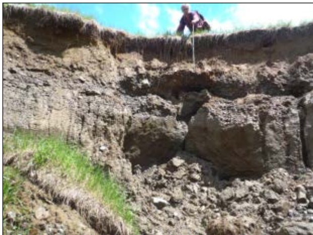
Figure 4. Upper fluvial sand and gravel (Unit A) exposed at head of landslide-gully complex at Cross Section A-A'.
