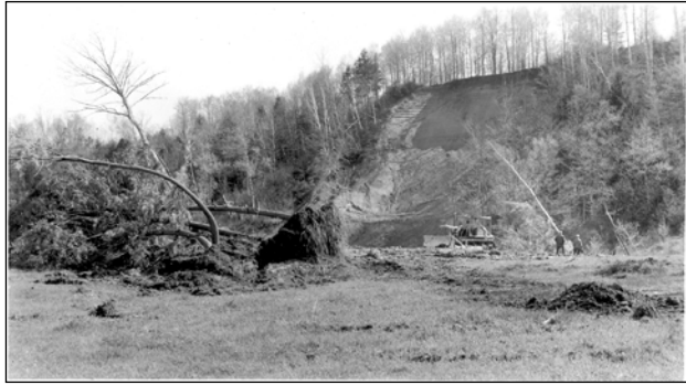
Figure 9. Landslide at site in May of 1954. Bulldozer for scale. The landslide occurred on the slope east of the river and is visible in the back, right. The trees in the foreground at left are part of the toe deposit and are on the west side of the river. Photo by Harold Thomas, from the collection of Wendell "Stub" Wells, Jeffersonville.
