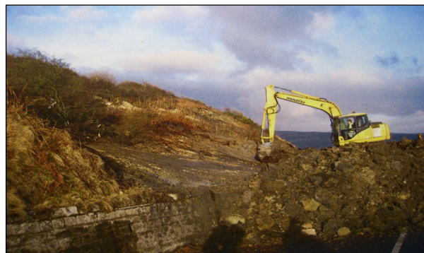
Figure 1. Landslide debris at Straidkilly on A2 Coast Road
