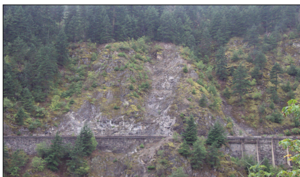
Figure 3. Cascade Rockfall site viewed from across the Fraser River from TLS scanning location
