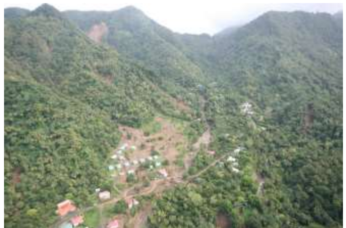
Figure 4. Debris flow at Fond St. Jacques during Hurricane Tomas (photo courtesy DFL Consult, Castries, Saint Lucia).
