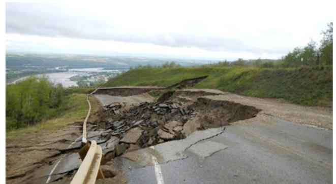
Figure 1 Landslide in northern Alberta near town of Peace River
