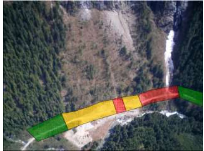
Figure 6: Subjective Probability of Rock Fall Over the 2 Year Construction Period. Low=Green, Medium=Yellow, High=Red
