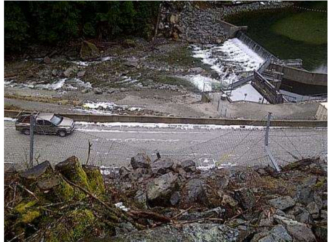
Figure 11: Rock Fence Damage as Viewed from Above
