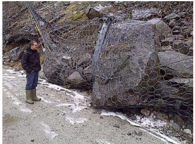
Figure 12: Rock Fence Damage at Road Level
