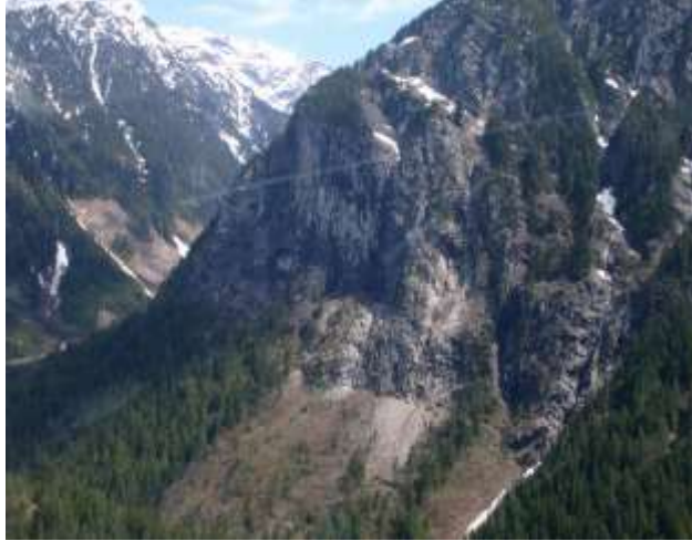
Figure 5: Overview of the Intake Location and Rock Fall Area
