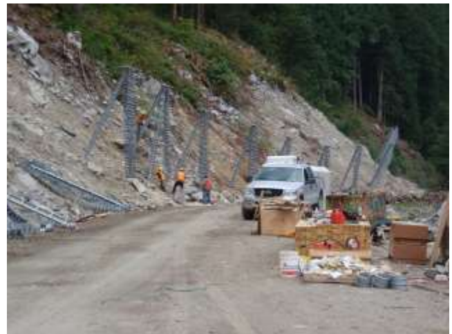
Figure 10: Installing the Fence Posts
