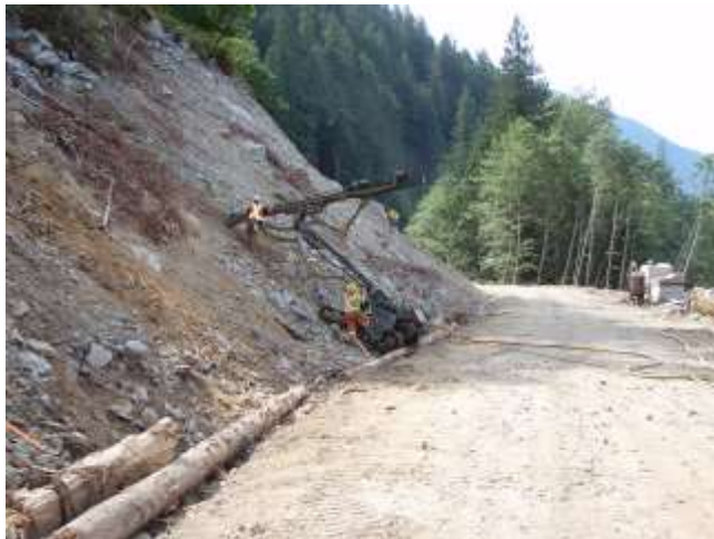
Figure 9: Drilling and Grouting for Fence Anchors
