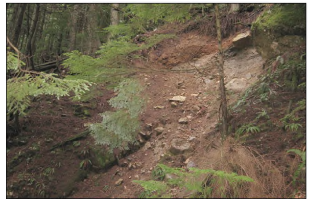
Photo 2. Looking upslope at a typical medium sized landslide that has deposited sediment and debris directly into the channel.
