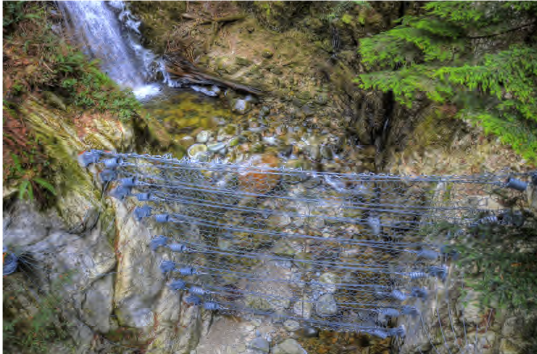
Photo 3. Looking upstream from above at the completed debris net located within the bedrock canyon.
