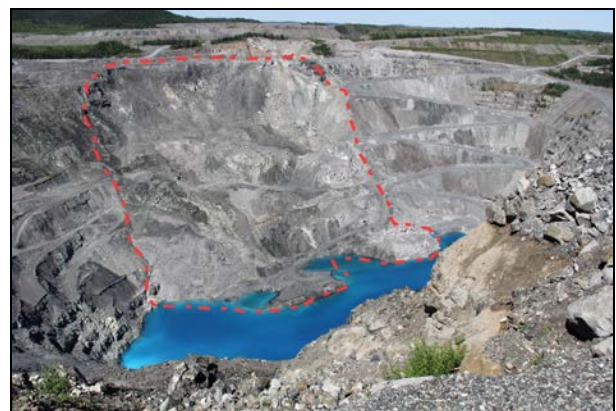
Figure 9. 2010 failure (red dashed line) in the West wall
