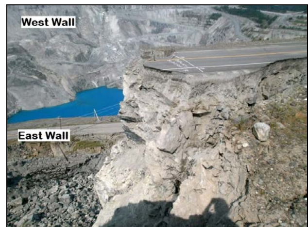
Figure 6. Failure of old highway 112 in the vicinity of the East wall (2012)
