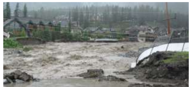
Figure 7. Upstream view of Cougar Creek from Elk Run Boulevard during the June 2013 flood.
