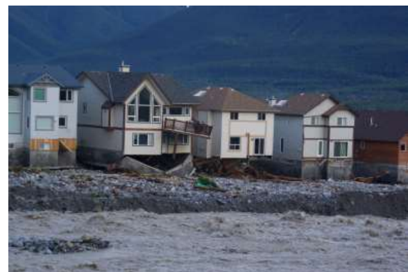
Figure 8. Damage to homes along left (east) bank of Cougar Creek between Elk Run Boulevard and Highway 1.
