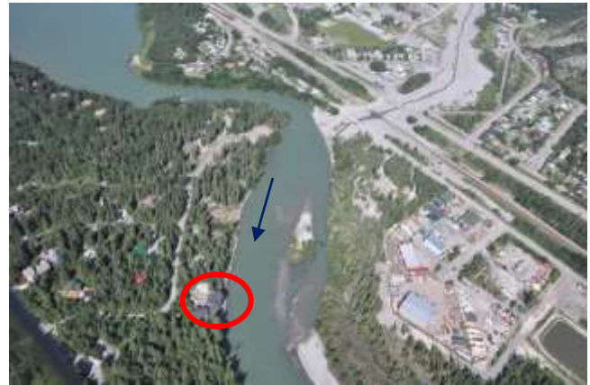
Figure 17. Aerial view of the confluence of Exshaw Creek with the Bow River. Deposition at the mouth of Exshaw Creek concentrated flows along the right bank of the Bow River, resulting in bank erosion and undermining of one home (circled in red). All homes of Lac des Arcs are located on Heart Creek fan.
