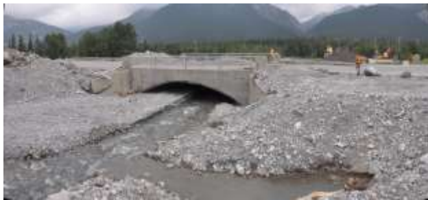
Figure 16. Downstream view of the Highway 1A bridge spanning Exshaw Creek. July 2013.
