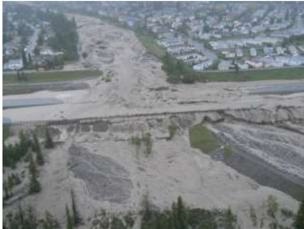
Figure 9. Lower Cougar Creek fan during July 19, 2013 flood. Photo: Alpine Helicopters.
