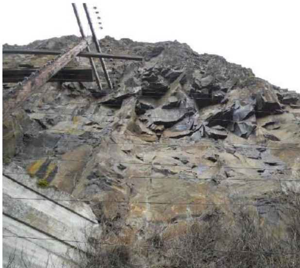
Figure 2. Photo showing the steep rock slope beside the railway tracks in the vicinity of the MRMS sensor Array 1.
