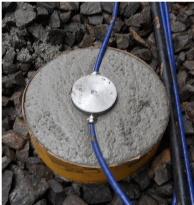
Figure 13. Each sensor was cemented in place to ensure good coupling to the ground and a horizontal orientation.
