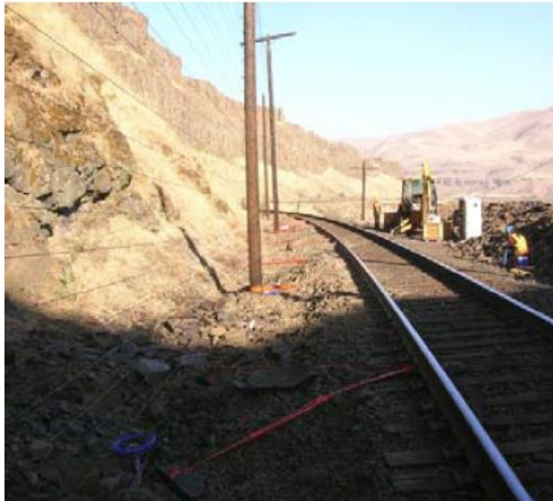
Figure 1. The location for Array 1. Microseismic sensors are installed at 5-8 feet from the railway track near to the location of the electric fence. The white box to the right is the location where the signals are collected and analyzed.
