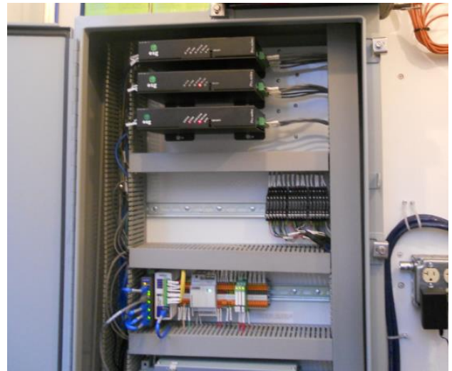
Figure 14. Photo showing the MRMS junction box inside the railway hut. Signals from the sensors are continuously digitized and analyzed for potential alarms (certain trigger criteria). The system also performs regular checks of system health. A webrelay unit allows mechanical control over switches such as railway lights.
