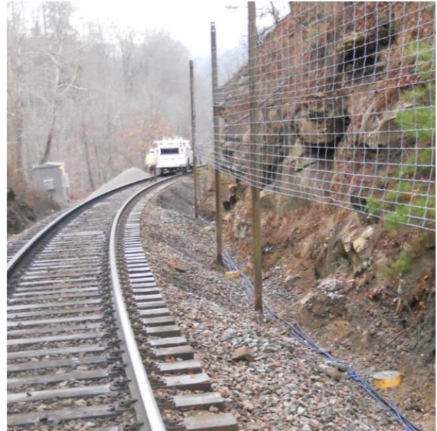
Figure 10. Photo identifying the location of some of the sensor for Array 2. The sensors are placed in a natural trench 5-8 feet from the railway line and near to the electric fence. The sensor cables pass through a conduit under the railway line and into the hut on the left of the figure where the digitization electronics is housed.
