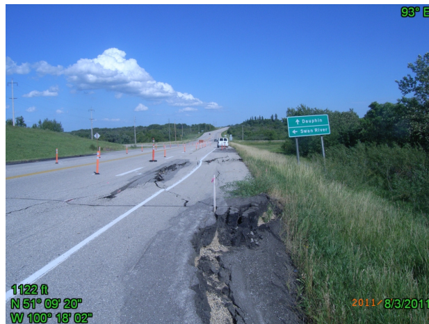
Figure 2. East on PTH 5 - Cracked Pavement Surface
