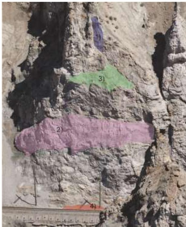
Figure 3: Gigapixel image of the site identifying characteristic areas: 1) Bedrock Material and Source Area; 2) Ledge features; 3) Talus Accumulations; and (4) Ditches. The non-coloured area was modelled as bedrock or was outside the scope of the model.
