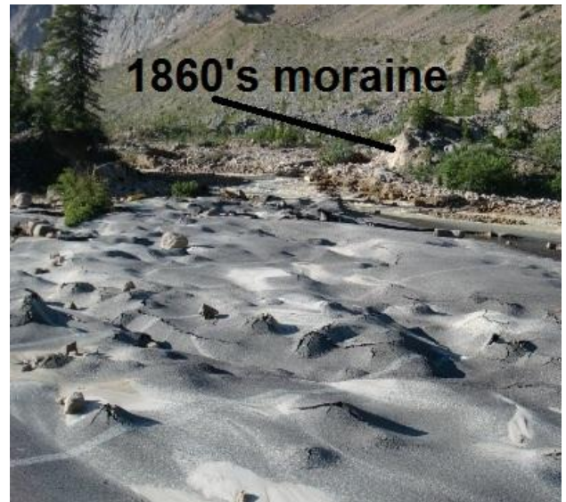
Figure 7 This August 11 th image shows the collapsed pavement in the parking area, undermined by erosion of the underlying fine material, resulting in its curious deflated appearance. (Parks Canada R.Wedgwood)
