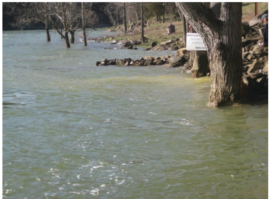
Figure 5. Dyed grout coming out into the river. This was a single occurrence and grouting was immediately stopped.
