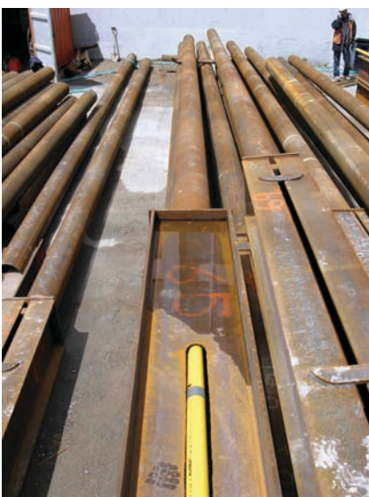
Figure 1. Lower section of pile with inclinometer casing transition to pipe pile.
