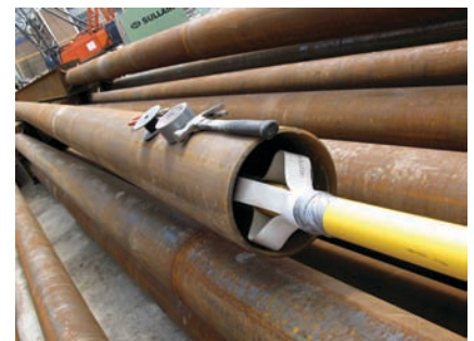
Figure 2. Centralizers in pipe pile section.
