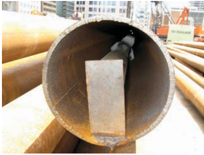
Figure 3. Custom welded inclinometer base.
