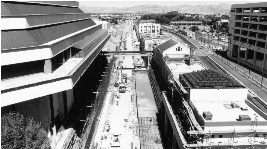
Figure 1. The ReTRAC rail trench is up to 33 feet deep, abutting sensitive buildings in downtown Reno, Nevada
