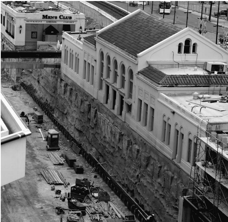
Figure 2. The historic Amtrak Station and Men's Club were two of the structures underpinned along the trench alignment
