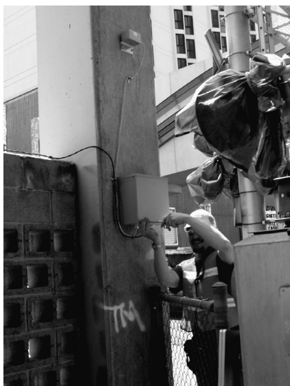
Figure 3. Typical ReTRAC instrument installation; tiltmeter is located on column above weatherproof enclosure containing step-down transformer and Wi-Fi transmitter.
