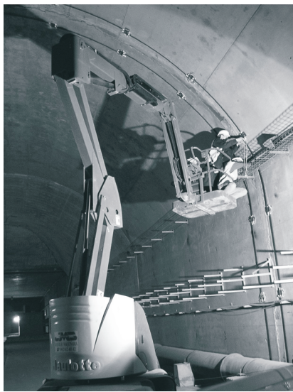
Figure 3. Installation of the Smart Rod.
