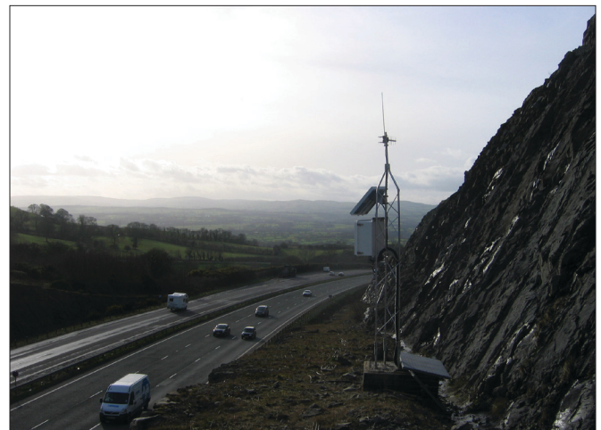
Figure 2. Photograph of the equipment installed at Rhualt Hill cutting.
