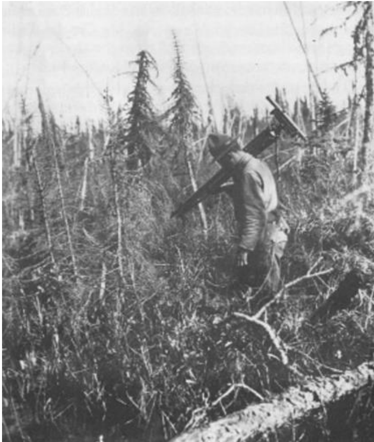
Charles surveying along HBR near KP 450, date unknown (source Eira Friesen, via Engineers and Geoscientists Manitoba)
