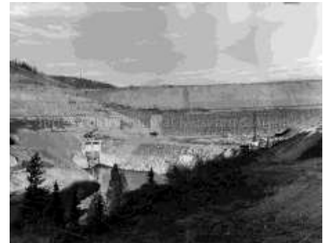
Kenney Dam construction, October 1952. Kitimat Museum photo #00016.
