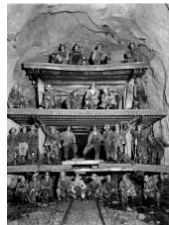
West Tahtsa main bore, part of the Kemano tunnel, March 1953. Kitimat Museum photo #00035.
